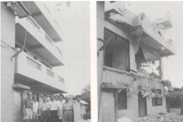
Before the demolition
